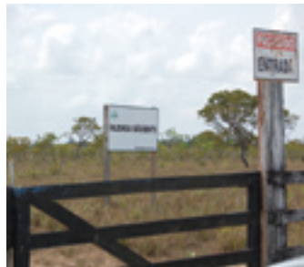
Preventing trespassers from entering by erecting railings and fences
