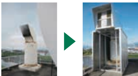
Before (left) and after (right) sound insulation measures have been implemented (Fuji Mill, Nippon Paper Industries)
