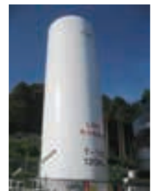
The LNG satellite facility installed at the Kochi Mill of Nippon Paper Papyrus
