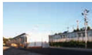
Temporary housing constructed on a company-owned site.
