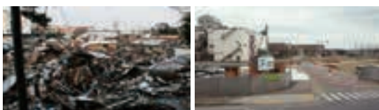
In front of Nippon Paper Industries' Ishinomaki Mill main gate in the immediate aftermath of the earthquake (left); An onsite photo taken on October 5, 2011 (right)
