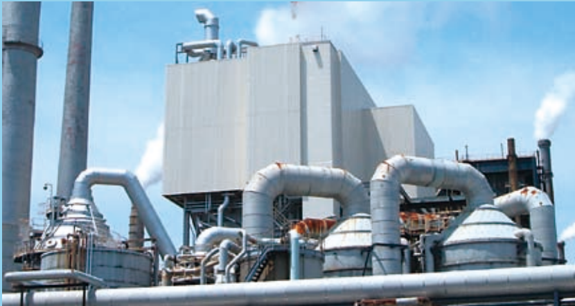
New energy boiler
