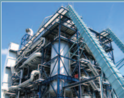
Biomass boiler (Nakoso Mill of Nippon Paper Industries Co., Ltd.)
