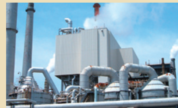
Biomass boilers at the Ishinomaki Mill
