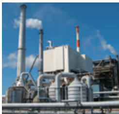
A biomass boiler at Iwakuni Mill
