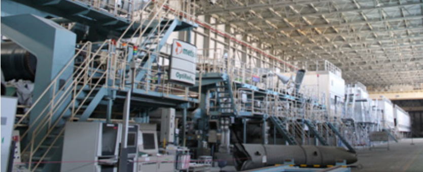
Paper machine on the 2nd floor (almost remained safe)
