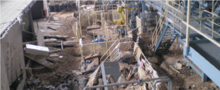
N6 packing machine on the 1st floor (heavily damaged)
