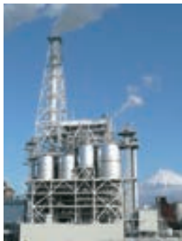
Biomass boiler No. 3 at Fuji Mill of Nippon Paper Industries
