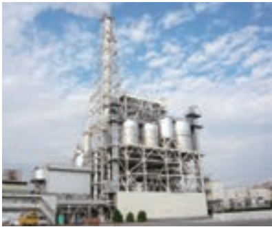
Biomass boiler No. 3 at the Fuji Mill
