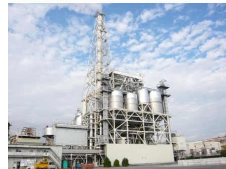
Biomass boiler No. 3 at Fuji Mill of Nippon Paper Industries
