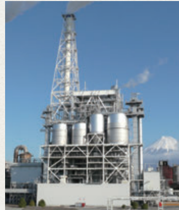
Biomass boiler already in operation (No. 3 Biomass Boiler at Nippon Paper Industries' Fuji Mill)
