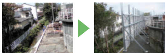
Before (left) and after (right) sound insulation measures have been implemented (Yatsushiro Mill, Nippon Paper Industries)
