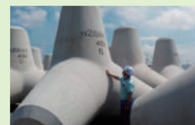
40-tonne breakwater tetrapod made with concrete containing CfFA®
