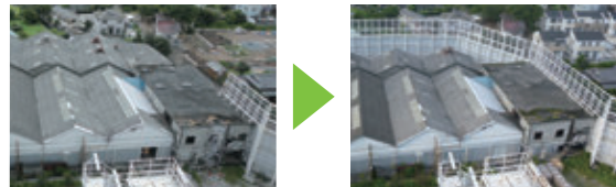
Before installation of sound insulation wall (left) and after (right) (Fuji Mill, Nippon Paper Industries)
