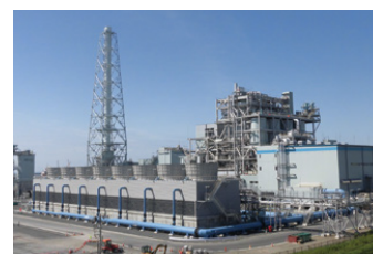
The biomass power generation facility at Ishinomaki Hibarino
