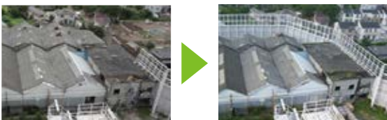
Before installation of sound insulation wall (left) and after (right) (Fuji Mill, Nippon Paper Industries)
