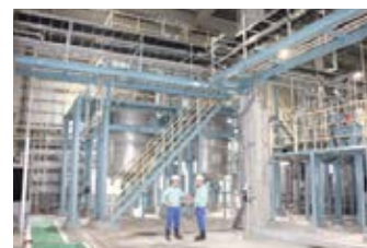
High-capacity production facility for CNF
