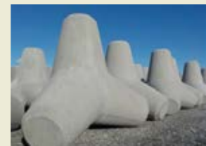
Breakwater tetrapods in a drainage outlet at Nippon Paper Industries Co., Ltd.'s Ishinomaki Mill.
