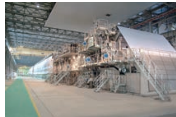
The N6 Machine at Ishinomaki Mill
