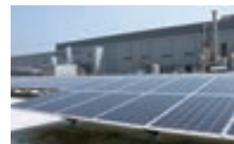
Otake Mill (Photovoltaic power plant)
