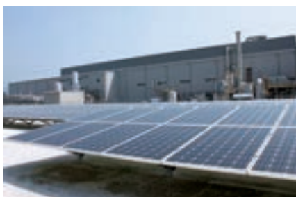
Photovoltaic equipment at Otake Mill
