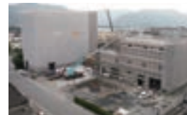
Yatsushiro Biomass Power Plant (under construction)
