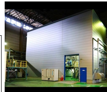
Hydrophobization facilities for raw pulp at the Fuji mill
