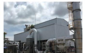
新規木質バイオマス燃料の実証設備(タイ) Demonstration facilities for the new woody biomass fuel (Thailand)
