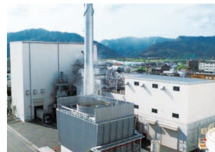
八代工場バイオマス発電所 所在地: 熊本県八代市 発電規模: 6,280kW 燃料: 間伐材等の未利用材100% The biomass power plant at Yatsushiro Mill Location: Yatsushiro City, Kumamoto Power generation output: 6,280kW Fuel: 100% unused woody materials derived from sources such as thinning wood
