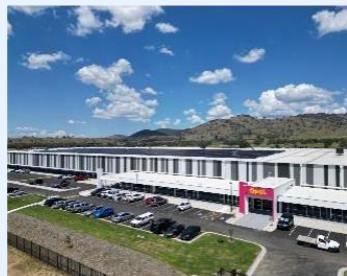
Wodonga Corrugated Box Plant (Operational since 2023)
