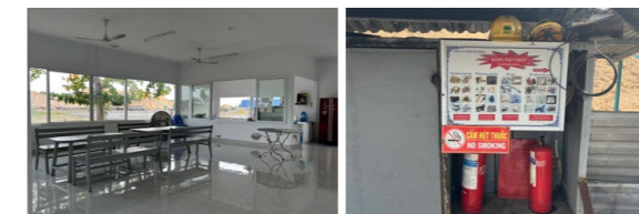
(Left) Clean break area equipped with air conditioning (Right) Fire extinguisher in chip yard and warning to prevent contamination
