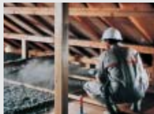
Installation of Insulation materials
