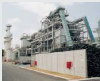
Boiler for waste power generation[*15] will contribute to cost reduction and reducing environmental impact: Nippon Daishowa Paperboard Tohoku Co., Ltd.
