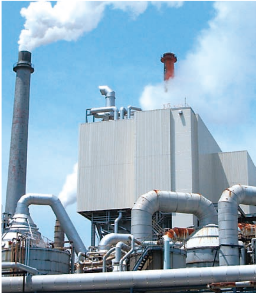
Biomass boiler at Nippon Paper Industries' Ishinomaki Mill
