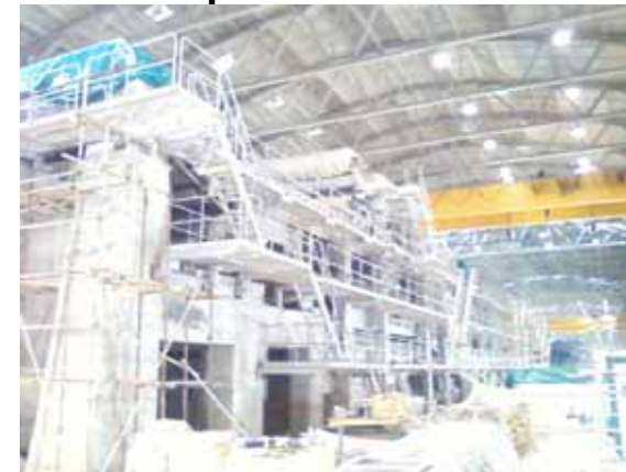
Coated duplex board machine being constructed at Hongmei Mill
