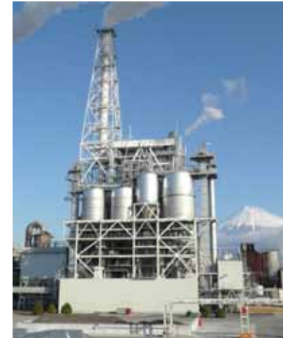
No. 3 biomass boiler at Nippon Paper Fuji Mill
