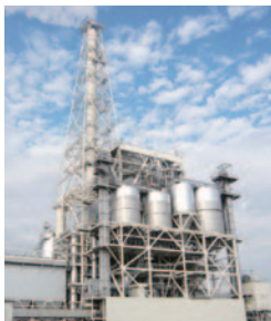
Fuji Mill No. 3 Biomass Boiler
