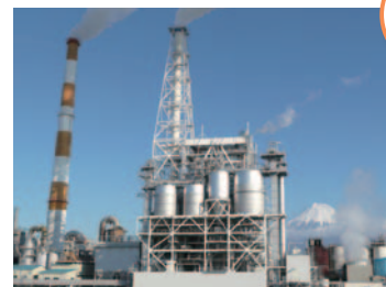
Power plant at Nippon Paper Industries Co., Ltd.'s Fuji Mill
