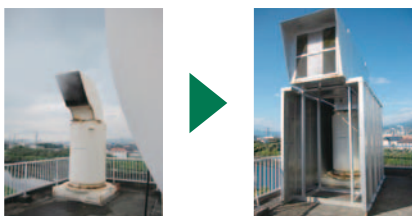
Before (left) and after (right) sound insulation measures have been implemented (Fuji Mill, Nippon Paper Industries)
