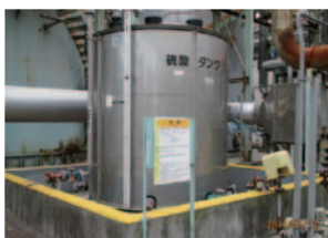
Liquid containment wall
