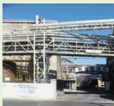
Cups are transported to NPI's Kanto Mill (Ashikaga)
