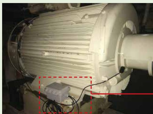
An e-wireless patrol device installed on an electric drive motor at Shiraioi Mill.
