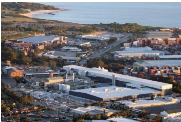
Opal Botany Mill (containerboard mill)
