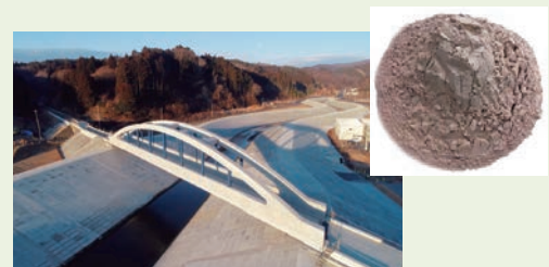
CfFA® was used in bridge beams, arches and vertical supports at the JR Kesenuma Line Sakuragawa Bridge on the JR Kesenuma Line (Minamisanriku Town, Motoyoshi District, Miyagi Prefecture)
