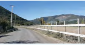
Fences installed by Volterra
