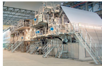
A paper machine that improved production efficiency
