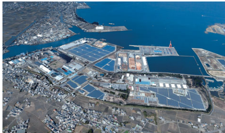
Komatsushima solar power generation facilities
