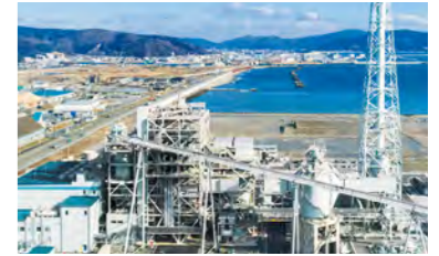
Ishinomaki Hibarino power plant
