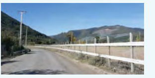
Fences installed by Volterra
