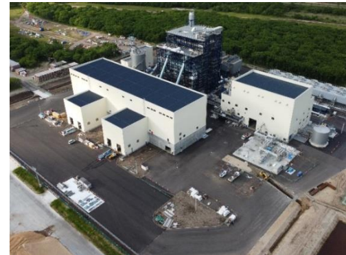
Yufutsu Energy Center, under constructing
