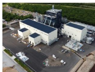
Yufutsu Energy Center, under constructing
