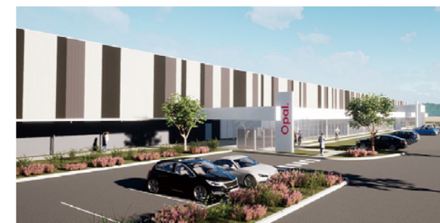
Conceptual image of the completed new corrugated box plant in Victoria, Australia
